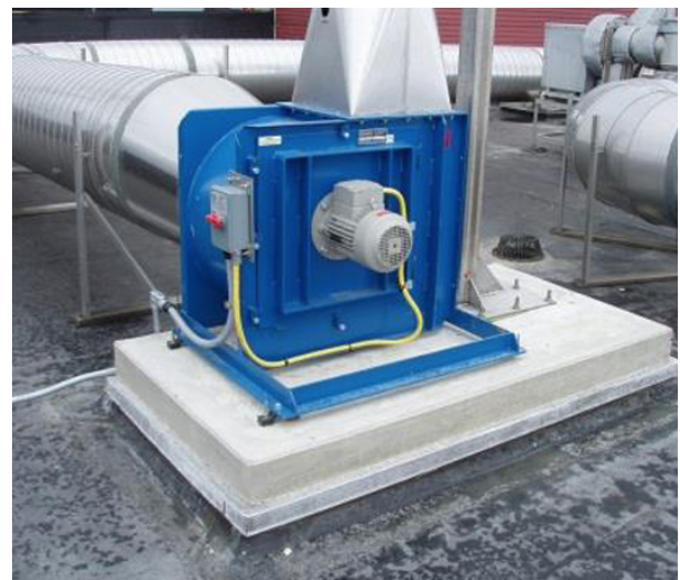
Fan placed on the roof.
