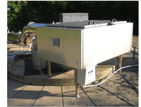
Jimco FLO-K air purification system installed by a Danish food manufacturer.
