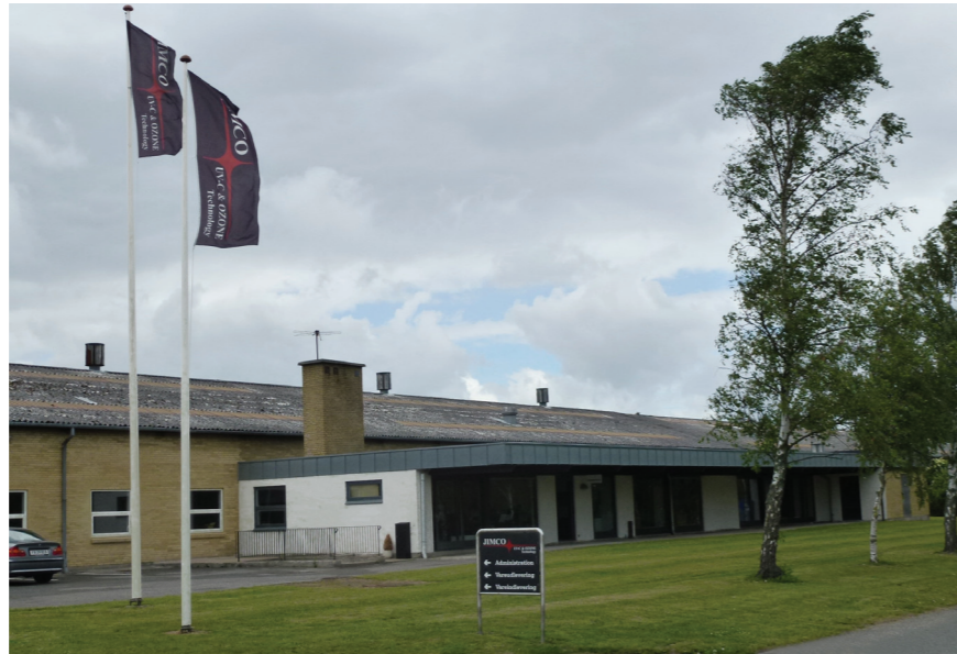
Jimco A/S headquarters in Rudkøbing, Denmark
